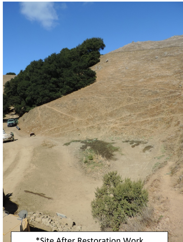
*Site After Restoration Work
